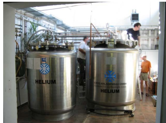
Fig. 2: Assembly of the 3000 litre LHe-dewar
